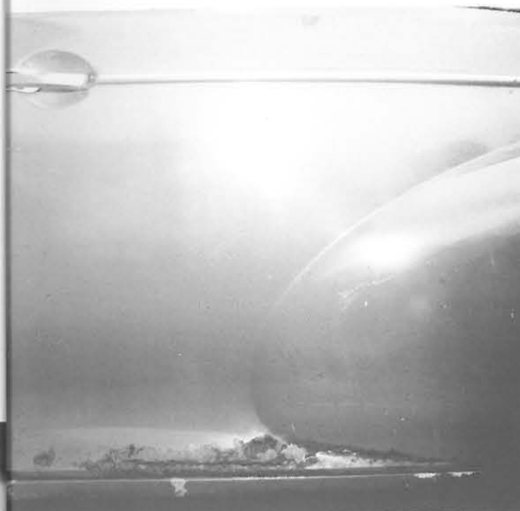
A rusty door which had been 'filled' again and again and painted at least 3 times after the first rust appeared.
